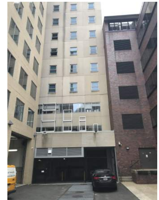
ALLEY LOOKING SOUTH
