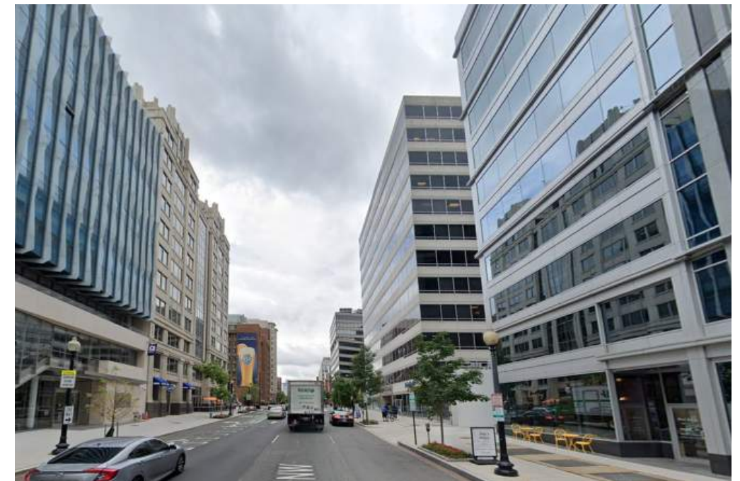
L STREET LOOKING EAST
